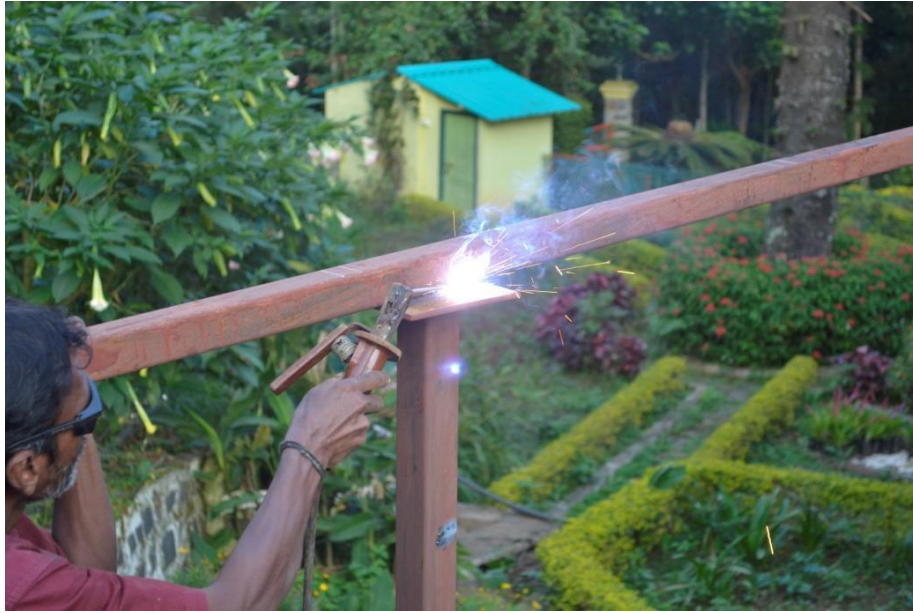
Welding work done while constructing the shed in the nursery
