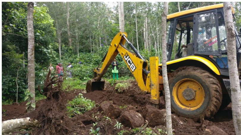
JCB Vehicle Clearing the stubborn bushes and stones to level the ground
