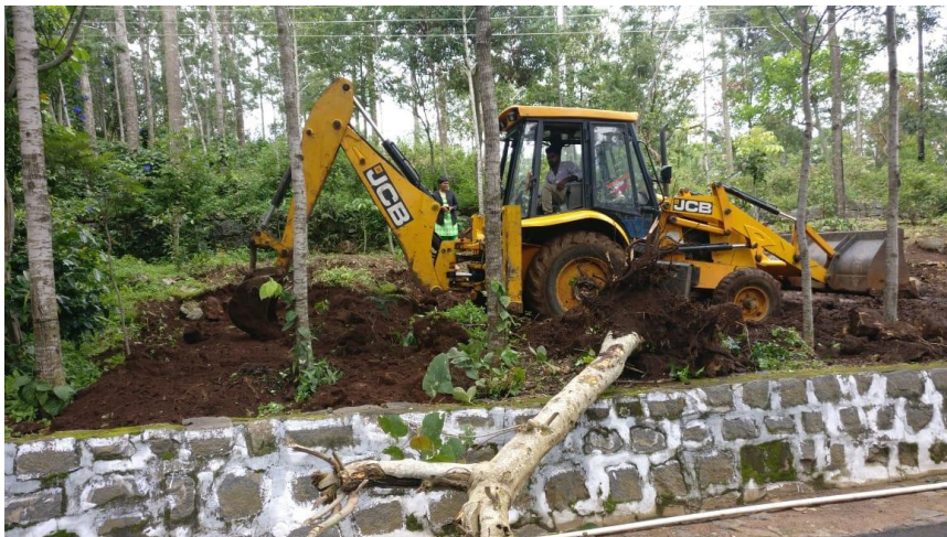
JCB Vehicle Clearing the stubborn bushes and stones to level the ground
